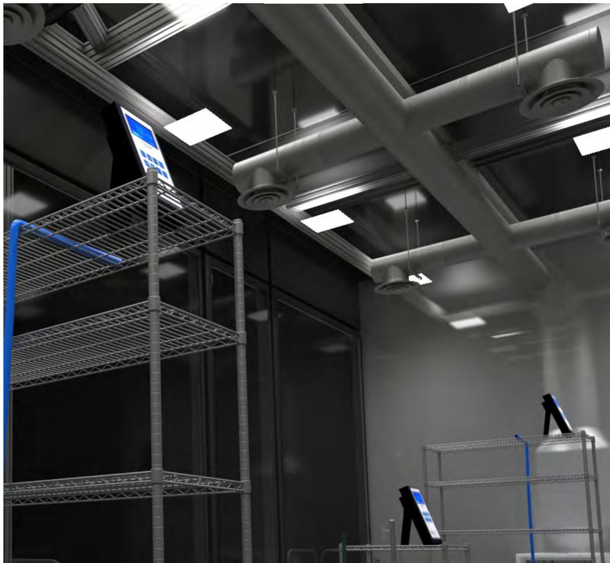
*Airborne ion concentration measurements should be logged at a point near air sampling ports being used for specific purposes, such as microorganism analysis.*
